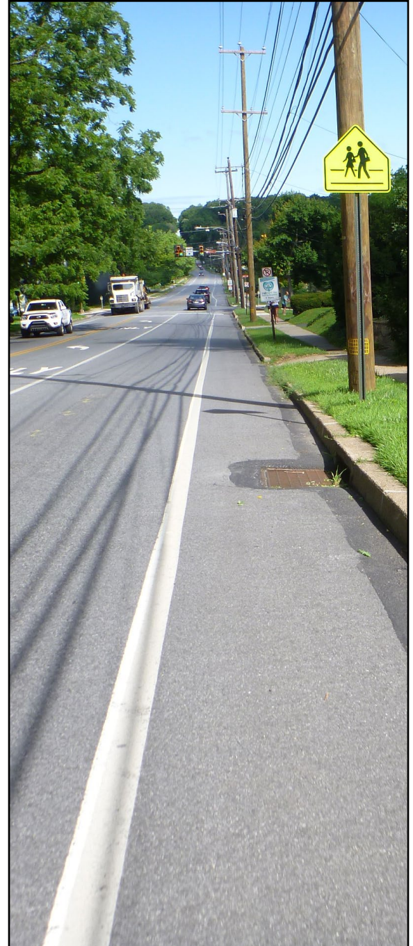
Susquehanna Avenue is an existing example of Class 2 Bikeway
